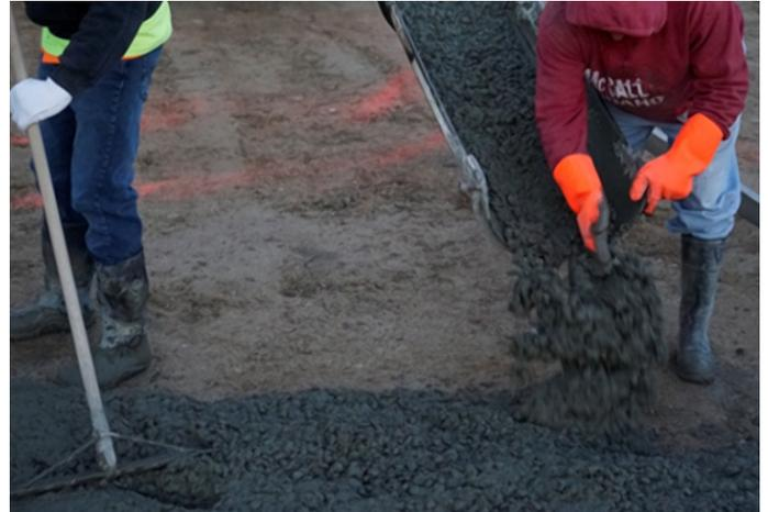
When cement is mixed with water a reaction occurs known as *hydration*.
